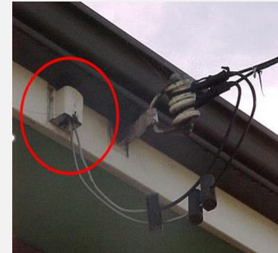
Image of Mains Connection Boxes and where they can be located
