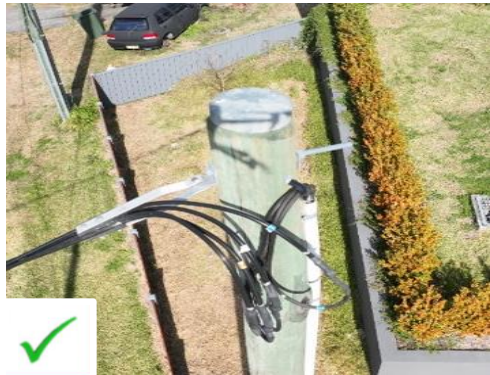
Image of 200Amp Service connected via Bolt and Lug
