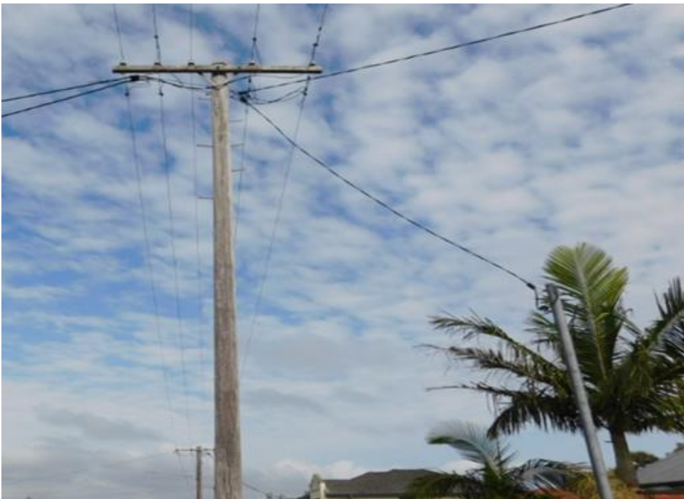
Image of Private pole A supplied via distribution mains pole
