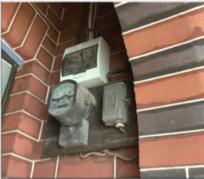
Image of metal clad service fuse
