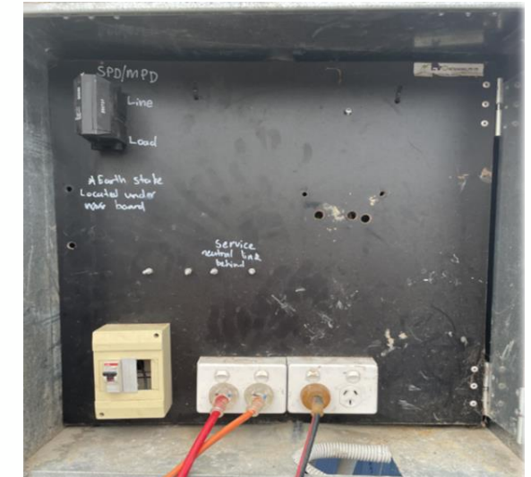
Image of Unmetered Supply
