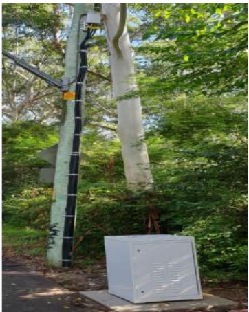
Small Cell Antenna with ground mounted equipment cabinet
