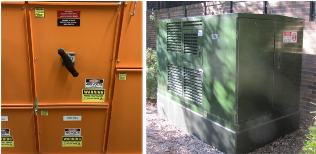
Image of Service protective device and kiosk substation
