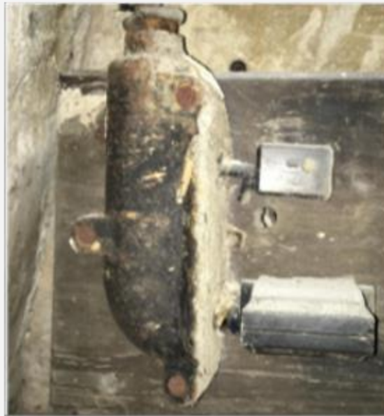
Images of metal clad service enclosures (handbag connections) with modifications completed
