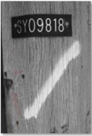
Image of Old defective pole marking
