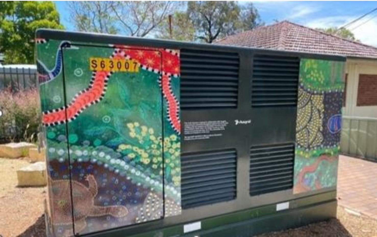
Image of Kiosk substation
