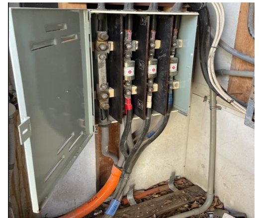
Image of metal clad service fuse cabinet
