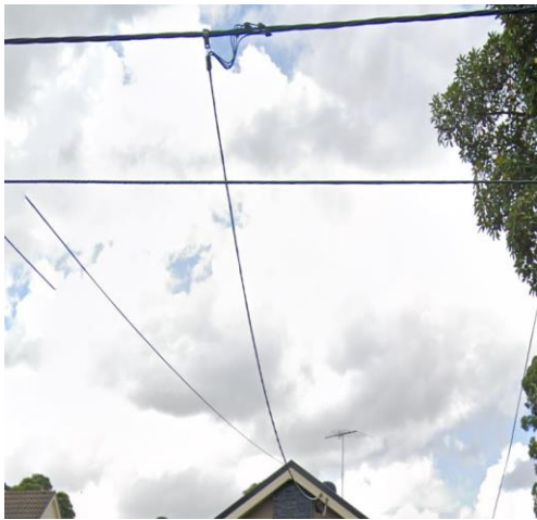
Images of Mid-span service from LVABC mains
