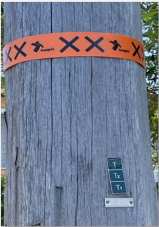
Image of Defective pole marking – Orange Band
