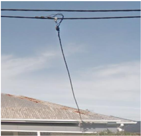
Images of Mid-span service from LVABC mains
