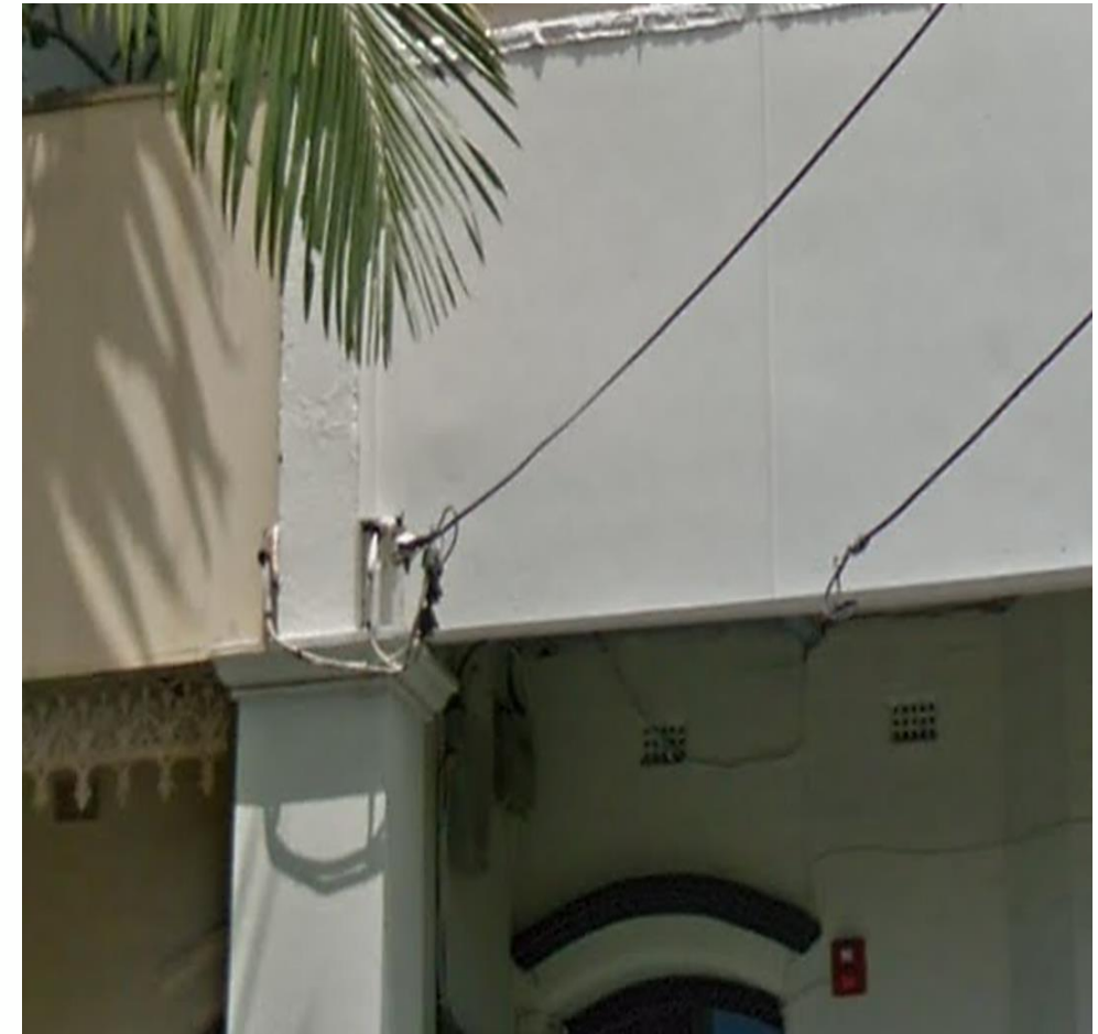
Image of Tap-off consumer mains connections
