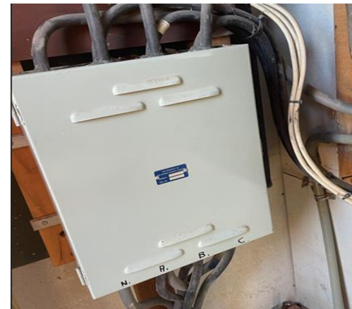
Image of metal clad service fuse cabinet
