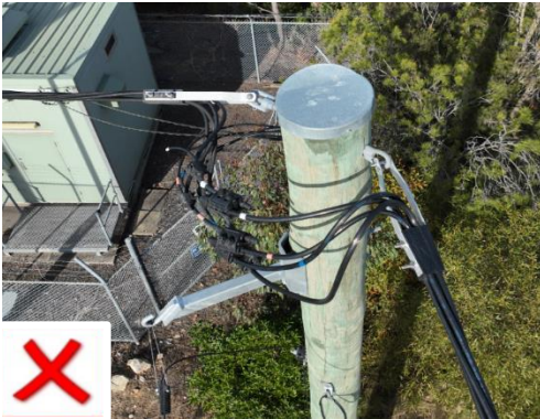
Image of 200Amp Service connected via IPC's
