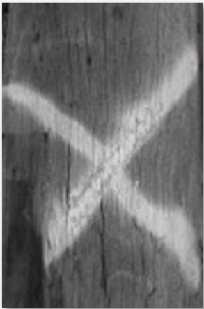
Image of Condemned pole cross
