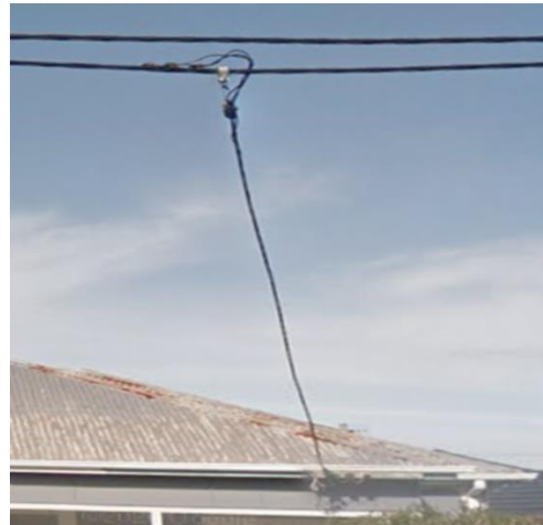
Images of Mid-span service from LVABC mains
