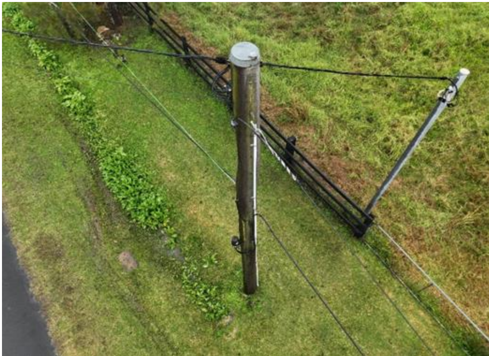
Image of Private pole A supplied via road-crossing pole
