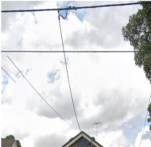
Images of Mid-span service from LVABC mains
