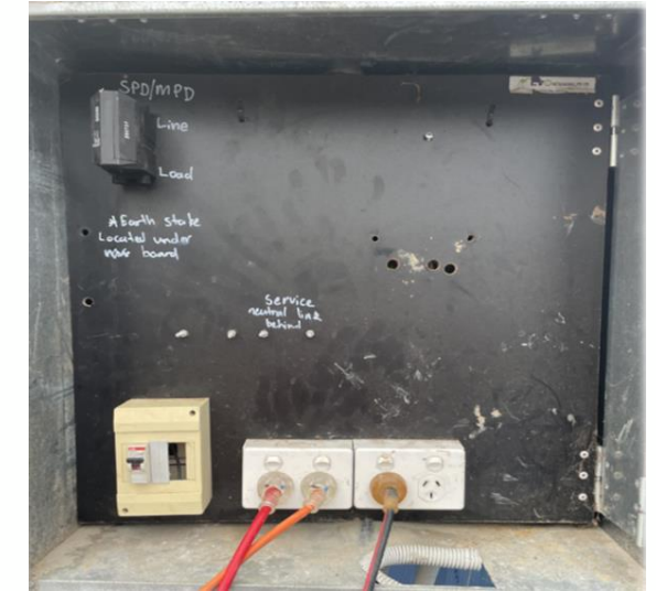
Image of Unmetered Supply
