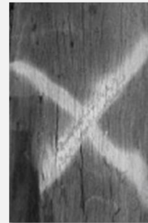
Image of Condemned pole cross
