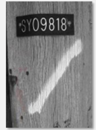
Image of Old defective pole marking
