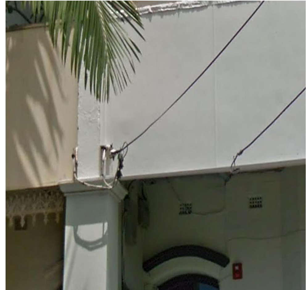
Image of Tap-off consumer mains connections
