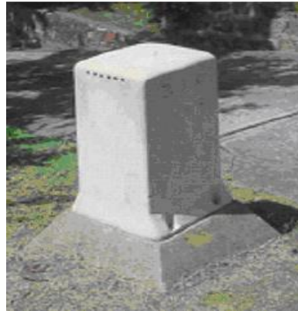
Image of Steel Framed Pillar
