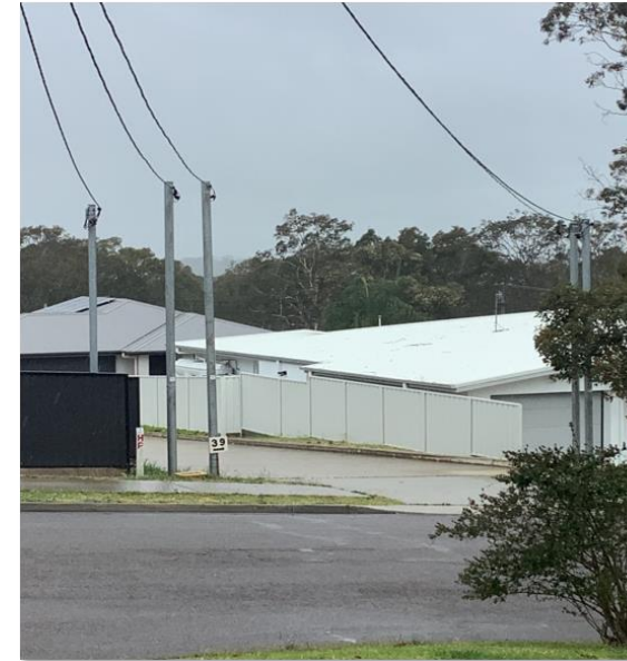
Image of Private poles installation on street
