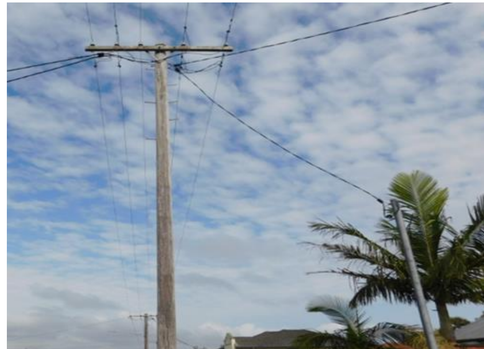
Image of Private pole A supplied via road-crossing pole
