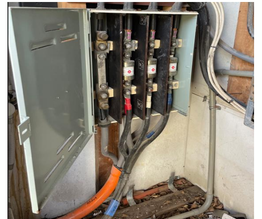
Image of metal clad service fuse cabinet
