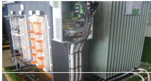
3. Remove 2 X M10 fixing bolts from R.H.S of galvanised channel base.
