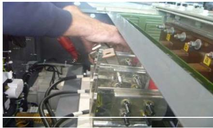
2. If DM&C equipment is installed remove wiring and fittings from the L/V Board.
