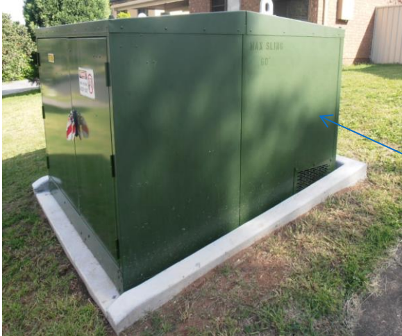
Padmount Square kiosk trial Muswellbrook NB: unable to cater for site slope
