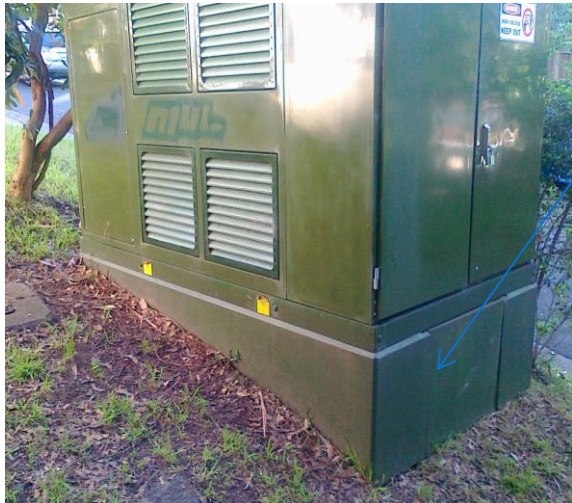
Typical sloping site install
