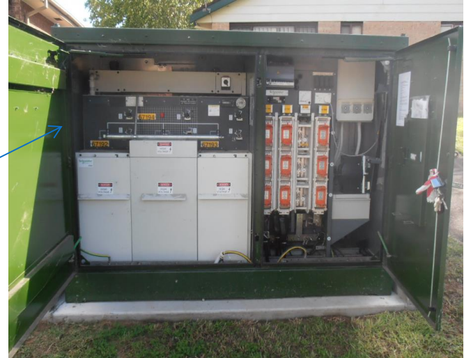
Padmount Square kiosk trial Muswellbrook NB: unable to cater for site slope
