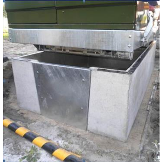
Kiosk installing on concrete tub
