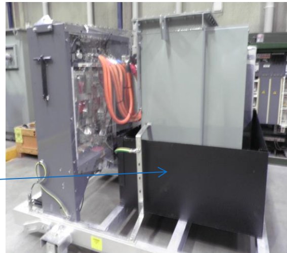
Typical internal padmount oil containment 'tub' stifles air flow and impacts ratings
