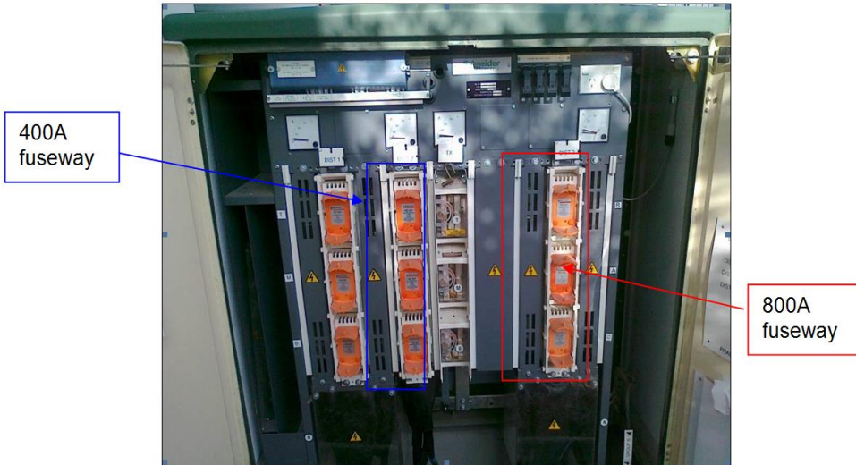
Typical SAIF Low Voltage Board 800A/400A/800A
