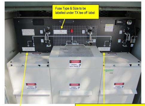
**RMI's**: All switches shall be labelled using laminated adhesive backed tape on white PVC sheet of minimum thickness 1.5 mm and nominal size 100 mm x 50 mm, or other size suitable for the equipment. Minimum letter height is 20 mm.
