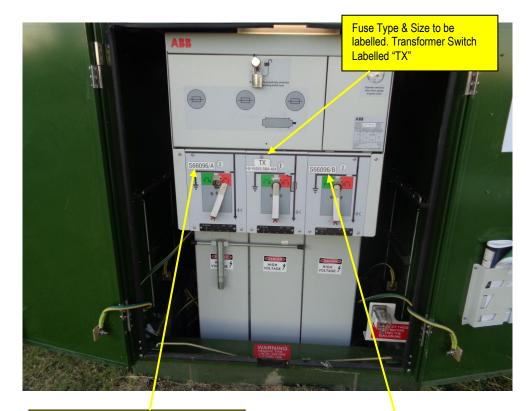
**RMI's:** All switches shall be labelled using laminated adhesive backed tape on white PVC sheet of minimum thickness 1.5 mm and nominal size 100 mm x 50 mm, or other size suitable for the equipment. Minimum letter height is 20 mm. These will need to be sourced and installed to this type of RMI utilizing suitable double sided tape.
