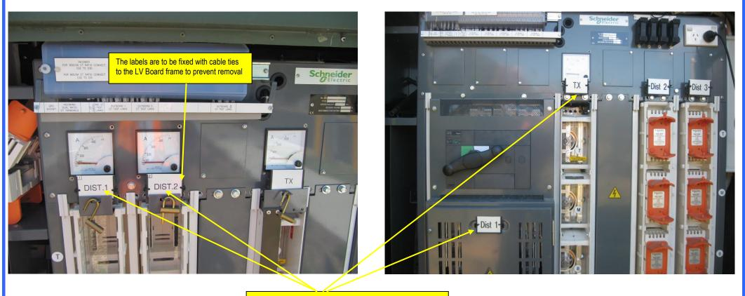
The number allocated to each distributor shall be attached beside the distributor control. Eg. Dist.1, Dist.2 or TX for Bus bar link
