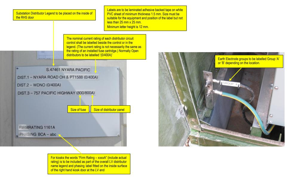
\*\*Please note for the Hunter region, the ASP is to place a Laminated LV diagram on the inside of the door in **addition to the legend** where the Distributor names are LVF numbers and are not descriptive of the LV destinations. \*\*
