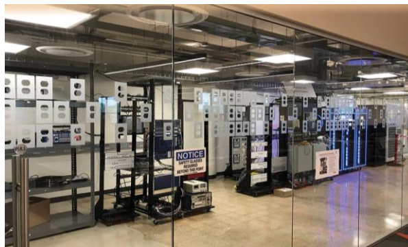
'Future grid' test lab – Chicago
