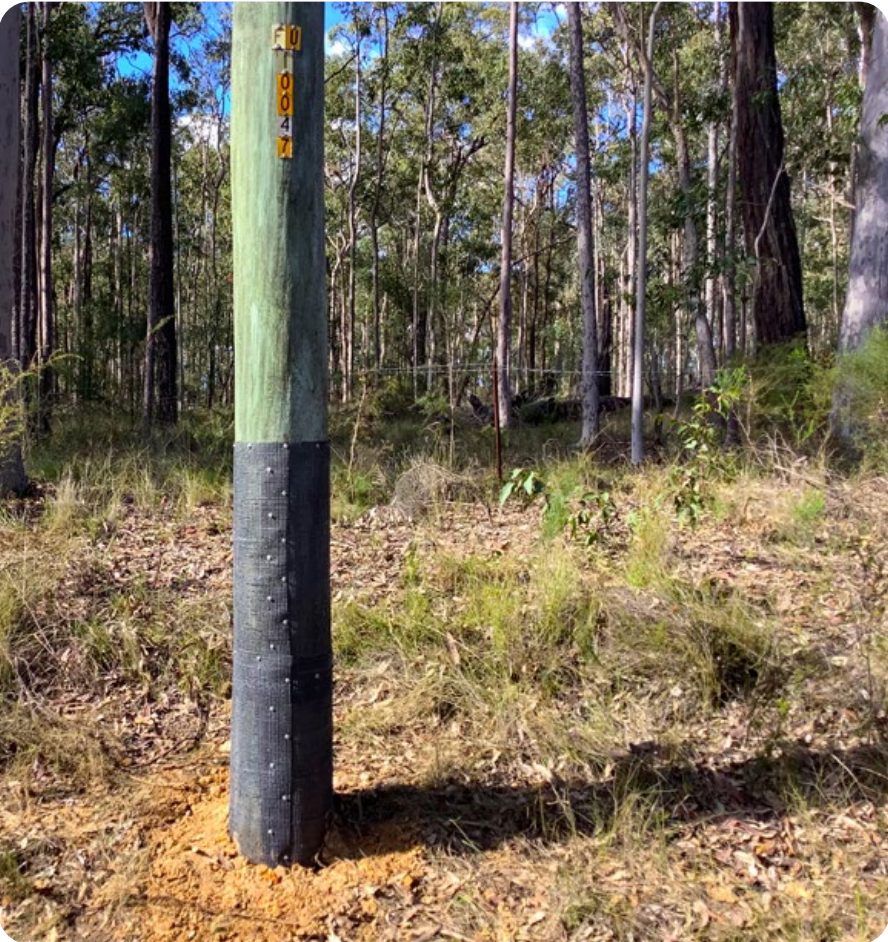
Fire Mesh fibreglass protection installed at the base of a timber pole.
