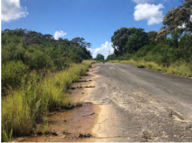
Figure 1 Ralston Avenue before works
