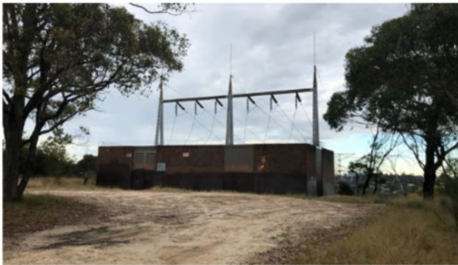
Figure 3 Western Lookout before works
