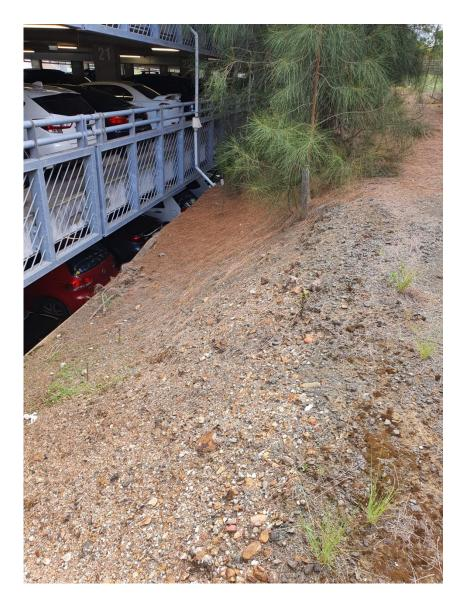
**Figure 5** - Image indicating the drop off from the raised level top of the berm and the steep sloping side-slope of the fill to the retaining wall about 1m below the crest.
