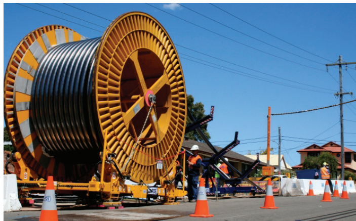
Cable installation on a similar project
