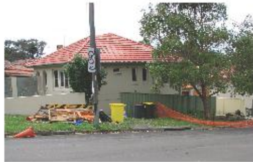
Poor housekeeping around work sites is a common cause of complaints.
