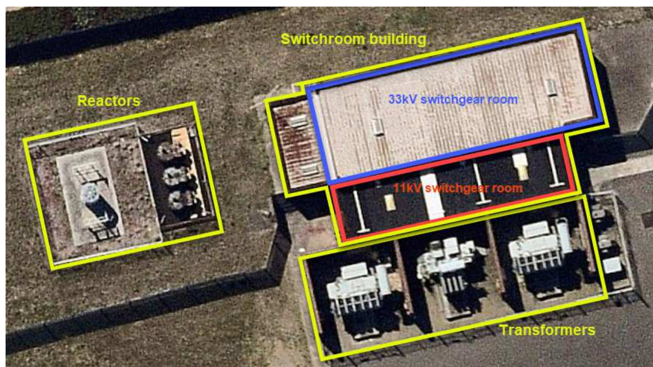
Figure 2.2 – Location of switchroom building at Sydney Airport zone substation
