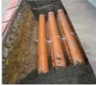
Open trench showing electrical conduits installed.
