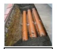
Open trench showing electrical conduits installed.
