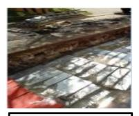
Cable trench with protective steel plates and orange PVC cover strip installed.
