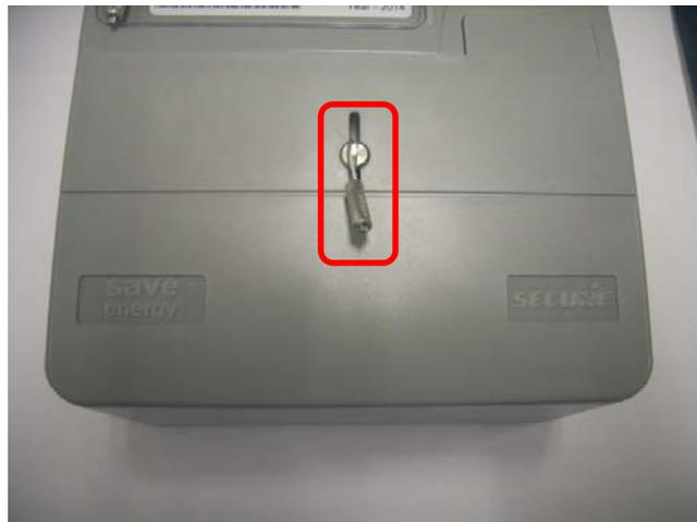
**Figure 8.4-8 Terminal Cover Seal after Installation**
