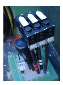
Figure 52 Single link – horizontally aligned
