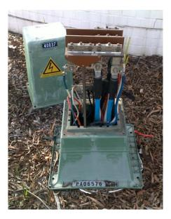
Figure 53 Double links – horizontally aligned
