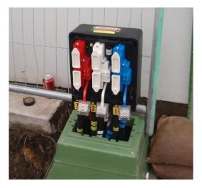
Figure 51 Double links - vertically aligned
