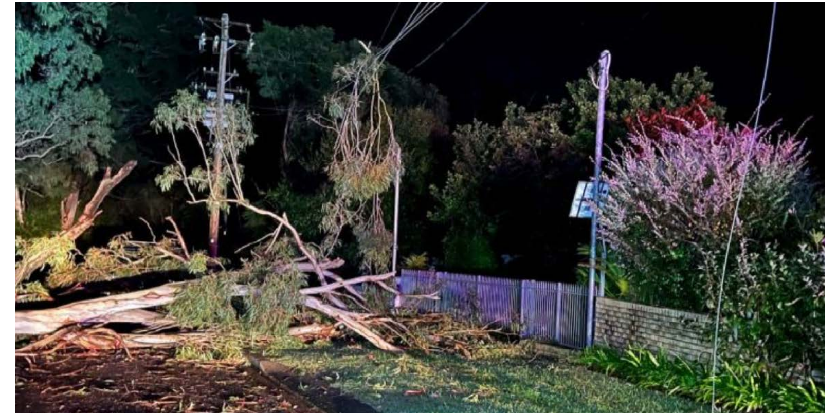
Storm damage in our network area.
